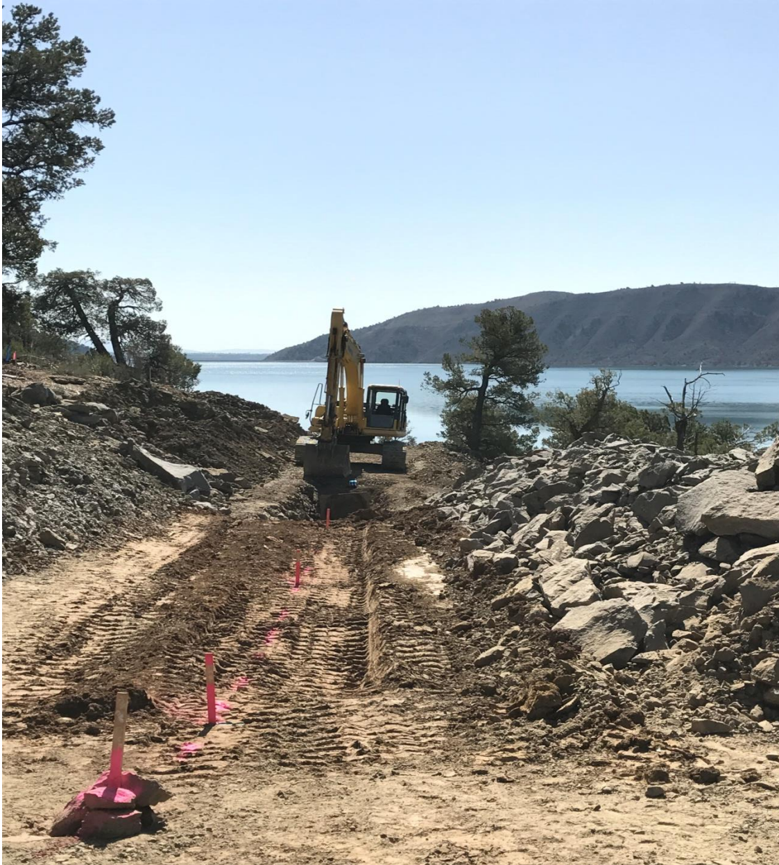
Figure 4: Constructed of 16 inch pipeline from Lake Nighthorse to Lake Durago
