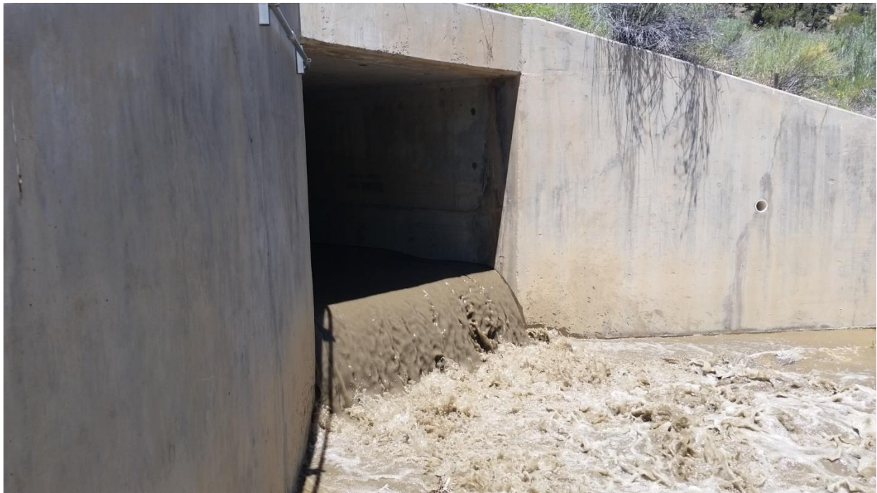
Figure 2: Box culvert on Basin Creek at La Posta Road
