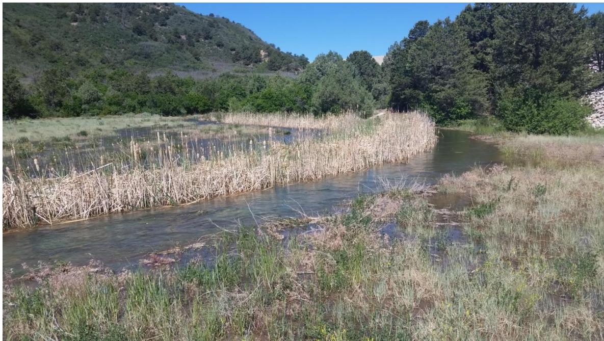
Figure 3: Constructed meandering channel on Basin Creek
