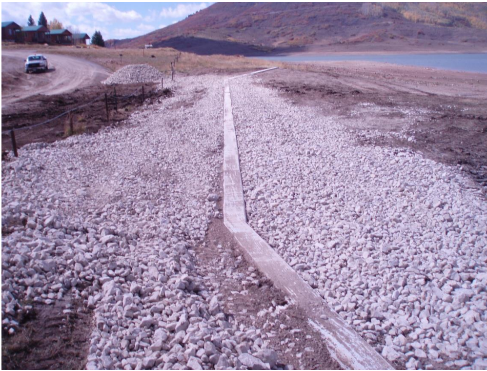
Figure 4: Groundhog Reservoir Grade Beam
