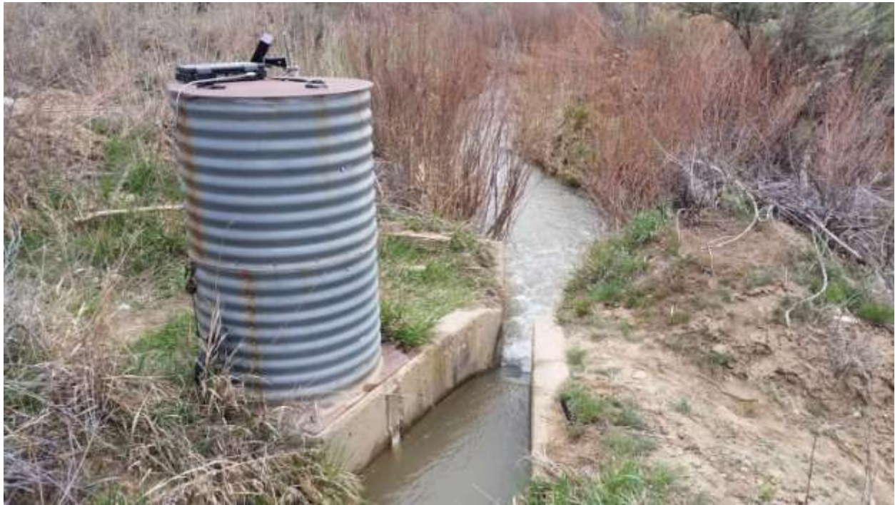
Figure 3: Pioneer Ditch flume to be relocated
