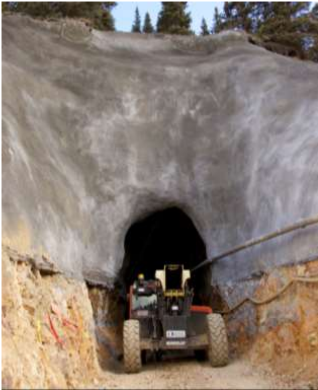
Figure 4: Gold King Mine entrance after discharge (November 2015)
