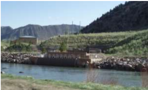
Animas-La Plata Project point of diversion and Pumping Plant
