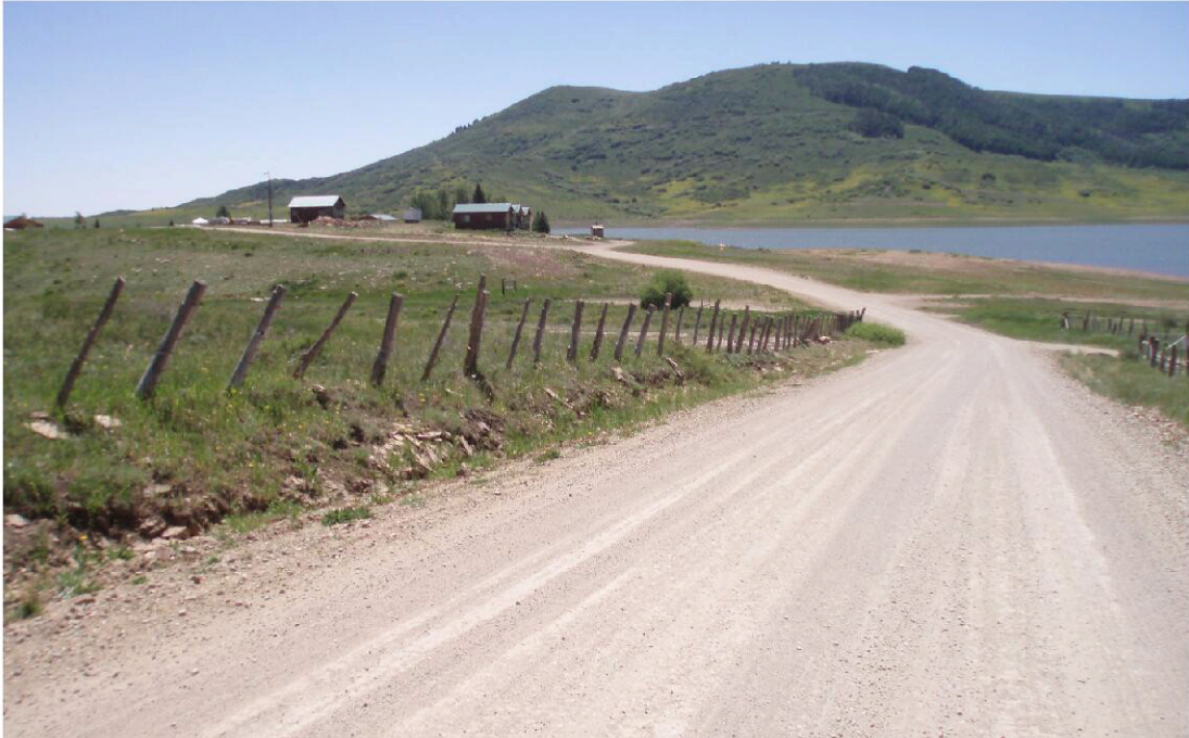
Photo of Groundhog Reservoir located in the Delores River drainage (District 71). The spillway crosses the road between the cabins and foreground. The roadway has been build up over the years due to wet conditions, thus raising the spillway elevation and causing dam safety concerns and additional storage. The dam is located just beyond the cabins out of view.
