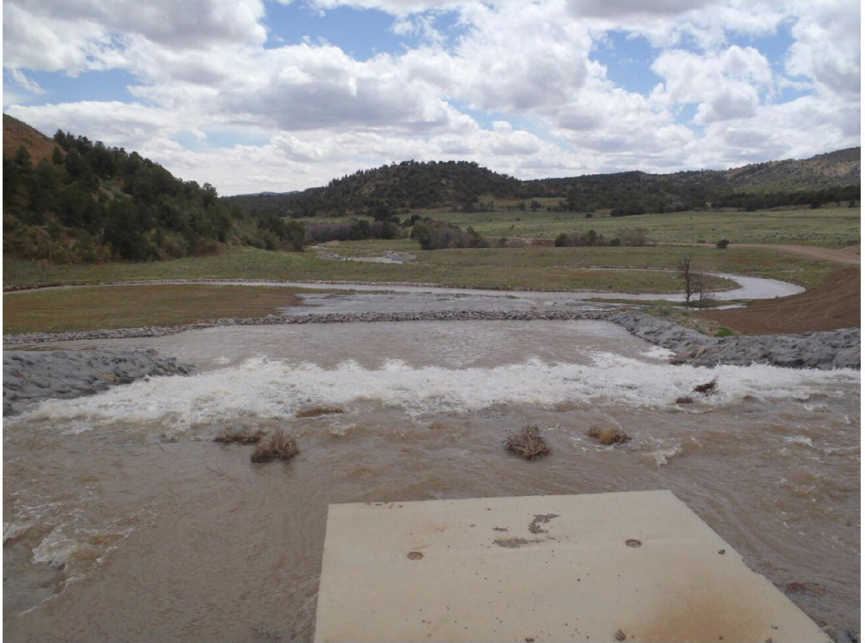
Constructed meandering channel in Basin Creek. Picture taken downstream of Lake Nighthorse (Animas-La Plata Project) during test release from reservoir.
