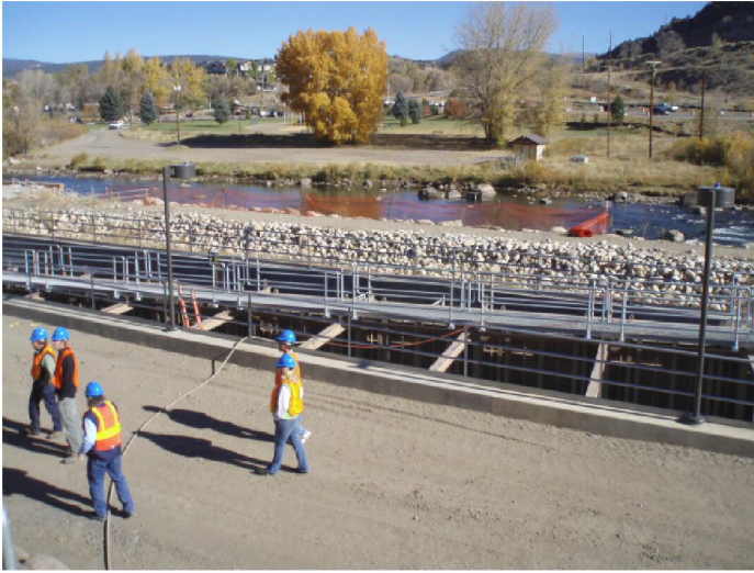
Outlet Structure in the bottom of Ridges Basin Reservoir, November 2008
