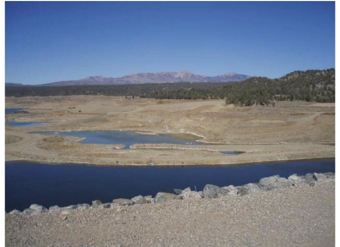
View from Top of Ridges Basin Dam of the La Plata Mountains, Water level should be about the tree line, November 2008
