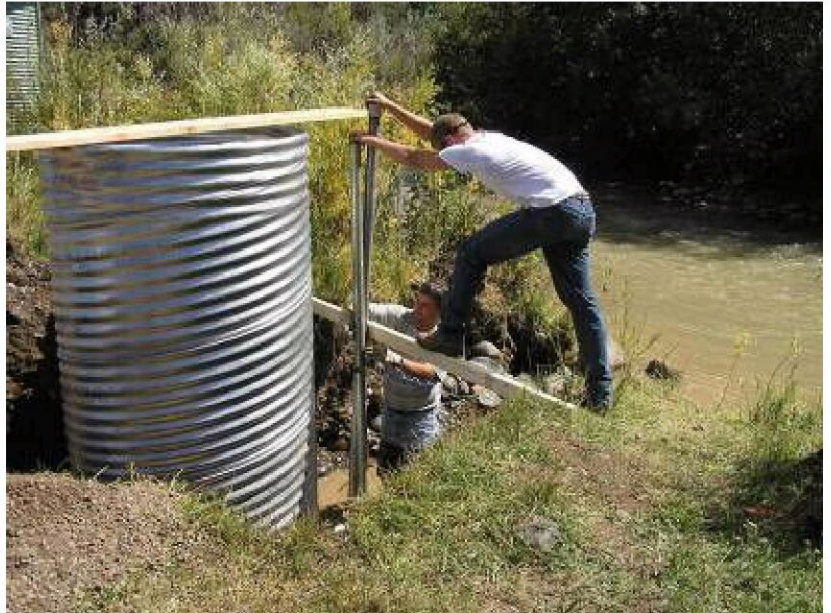
Brian Boughton, Hydrographer and Cheston Hart, EIT installing a new gage on the Lower Blanco River in July 2007.
