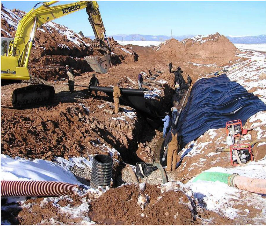
An inspection of construction for an Infiltration Gallery near the La Plata County Airport
