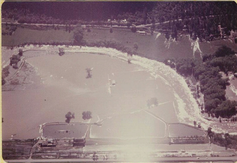
TURNER PONDS AND PUMP STATION (Four Miles North of Durango)
