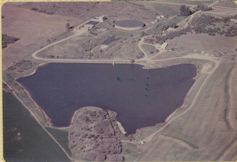
DURANGO REGULATORY RESERVOIR AND TREATMENT PLANT (College Hill)
