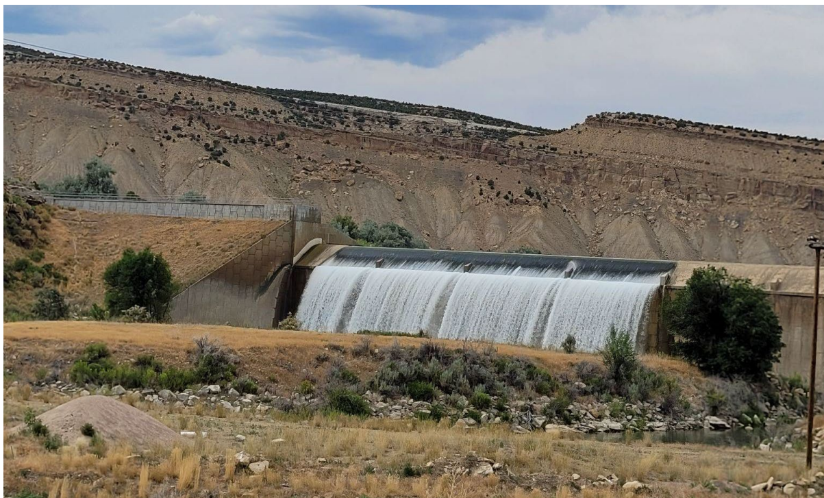
Taylor Draw Reservoir Spillway, Photo Credit: Betty Kracht
