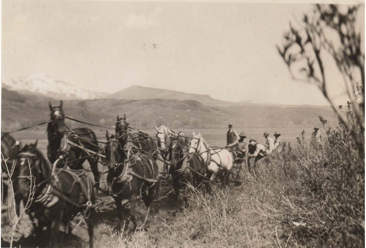
Construction of Keller Ditch, Appropriation date October 1, 1885
