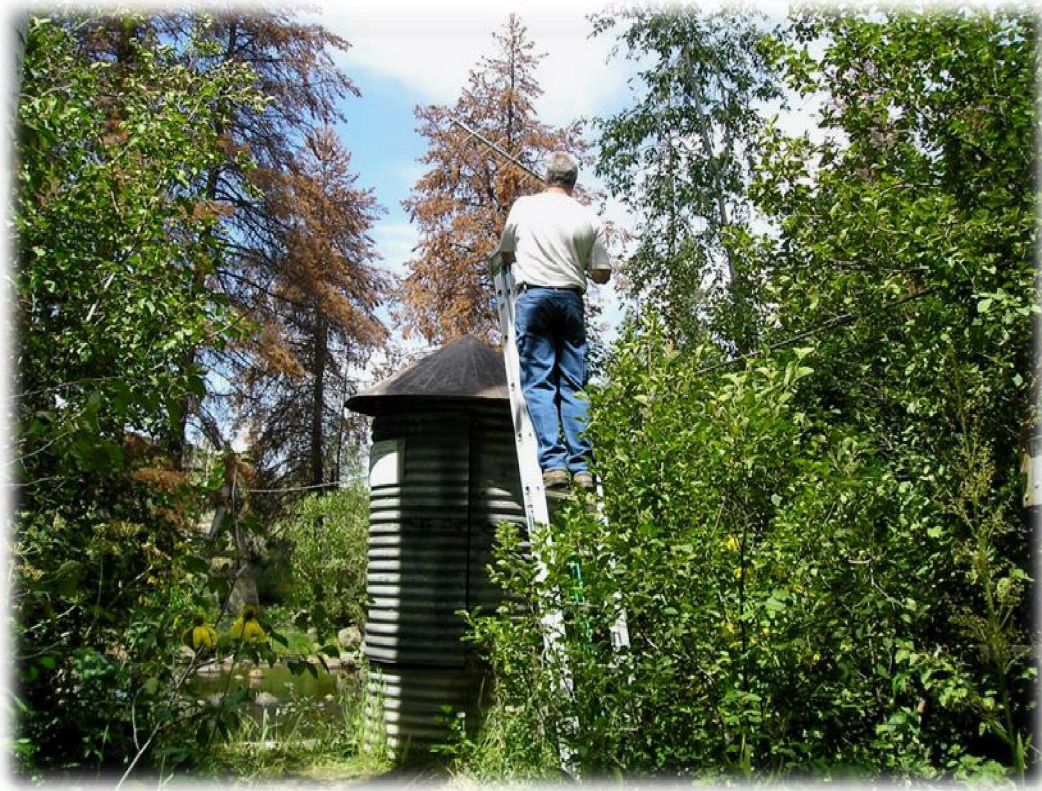
Installation of Solar Panel/Telemetry System at the Walton Creek Gage Station
