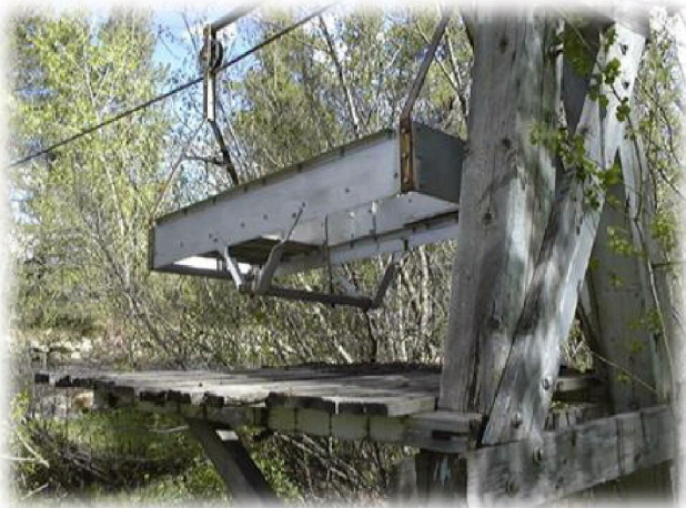
Condemned Cableway at Walton Creek
