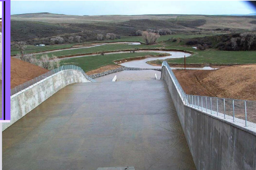
Elkhead Creek Reservoir Spillway
