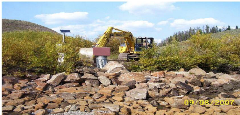
Gage Station Construction at Willow Creek below Steamboat Lake
