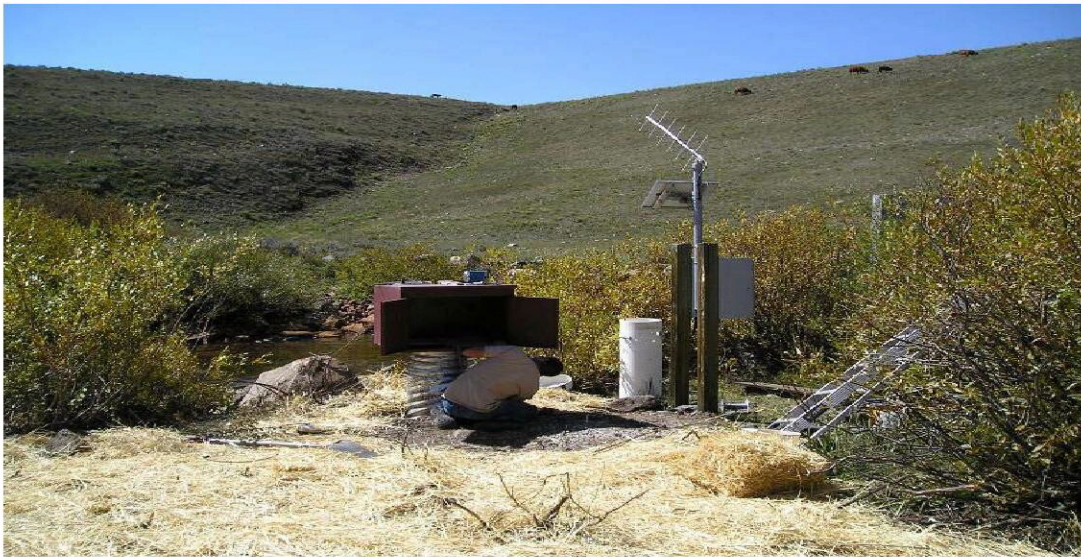
Improved Gage Station at Willow Creek below Steamboat Lake
