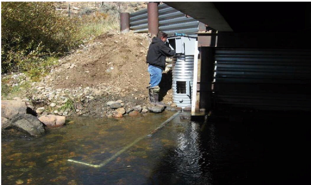
Upgrades to the Michigan River near Meadow Creek Gage Station
