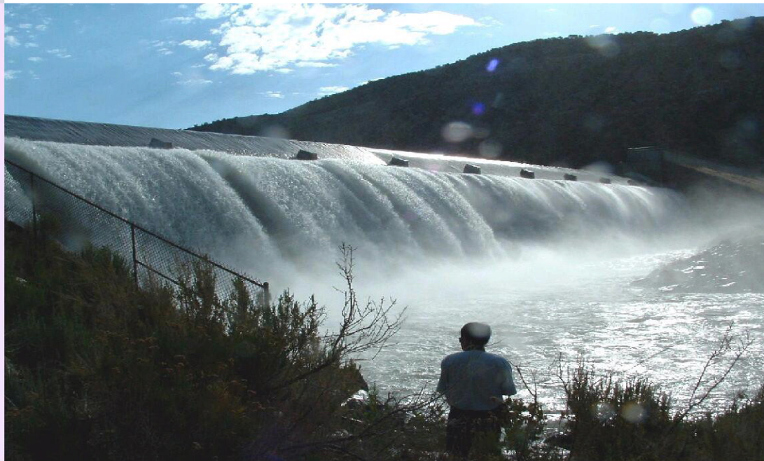
Taylor Draw Spillway
