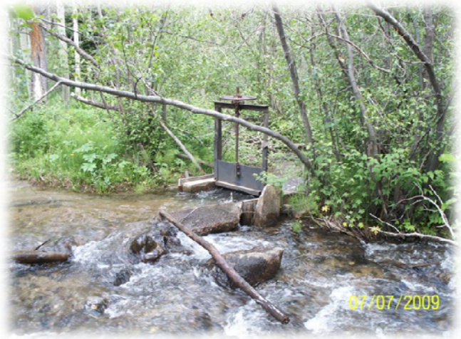
Carwood Ditch – WD 36
