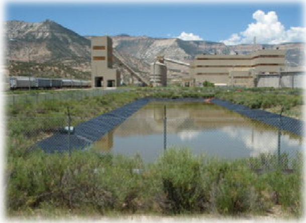
American Soda Storm Water Retention Pond – WD 39
