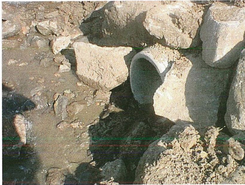
The downstream end of the new 24"RCP outlet at Mesa Creek #2.
