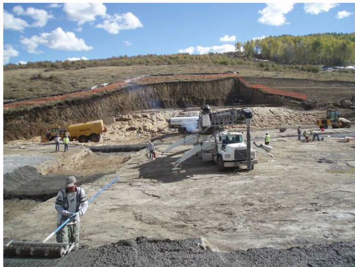
Foundation treatment at Cornerstone Dam
