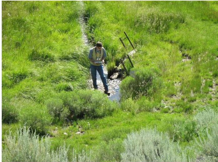
Jason Ward inspecting McDonough Dam #2.
