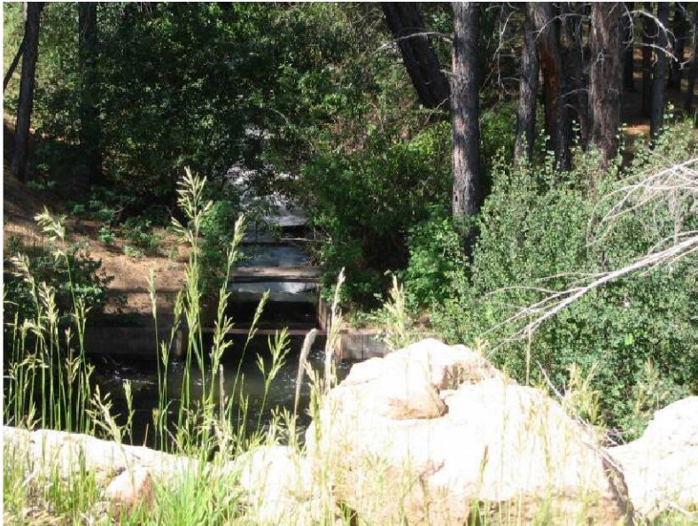
Flume on outlet of Buckeye Reservoir
