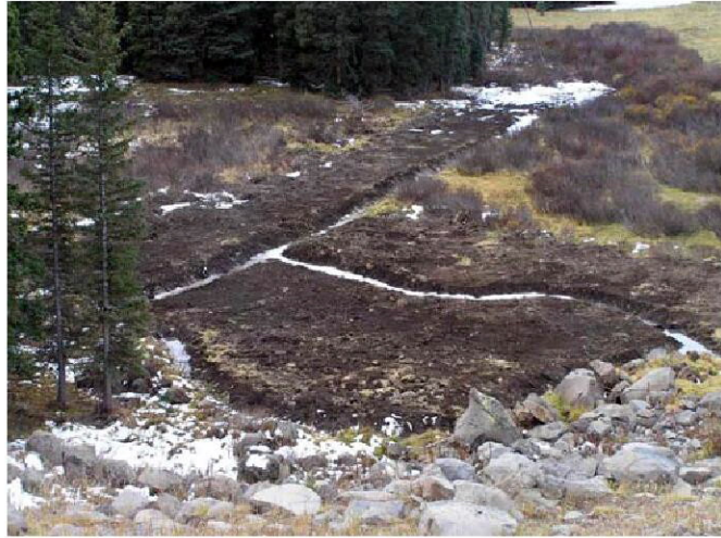
Youngs Creek Dam after repair
