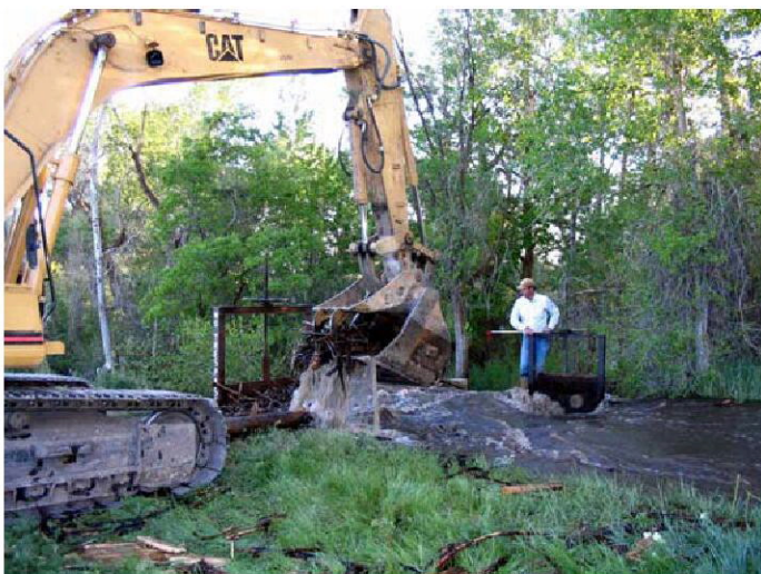
Surface Creek at Alfalfa Ditch Headgate
