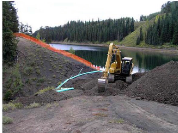
Meridian Lake Dam reconstruction
