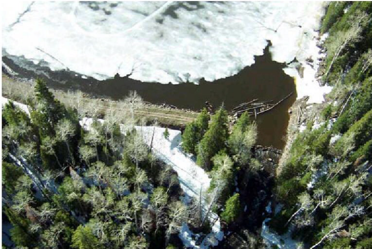
Aerial inspection of Grand Mesa spillway
