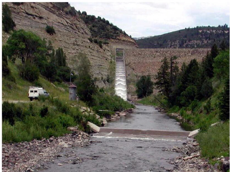
Ramp flume on Muddy Creek below Paonia Dam
