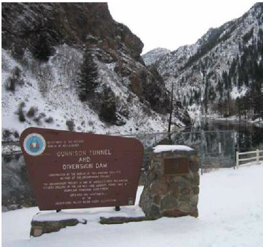
Gunnison Tunnel Diversion in Black Canyon
