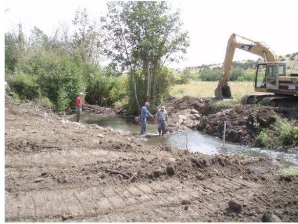
La Garita Creek Construction
