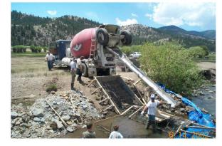
concrete weir had developed some small cracks in it over the last several years. During the very low flow periods this year, the entire flow of the stream was simply running through these small cracks, causing the gage to be isolated from the stream. Repair was made to the entire control. This repair should allow the control to operate properly for many years to come.
