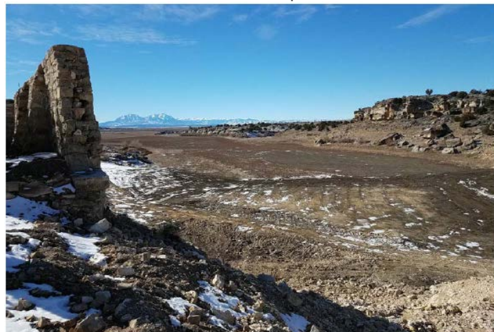
Looking upstream from dam through reservoir
