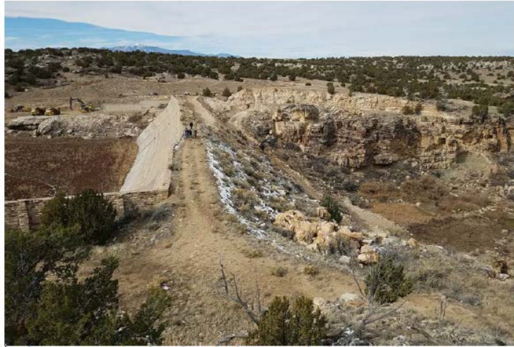
Dam prior to removal
