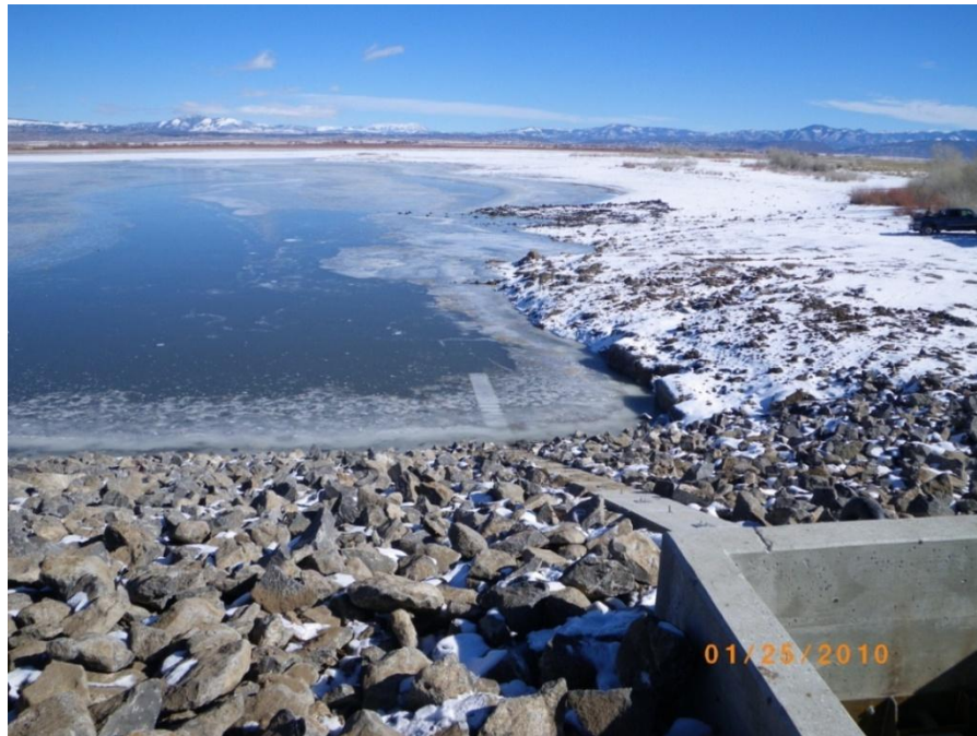
Smith Dam after upstream slope and outlet repairs were completed.
