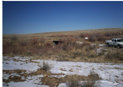
Overview of Site
