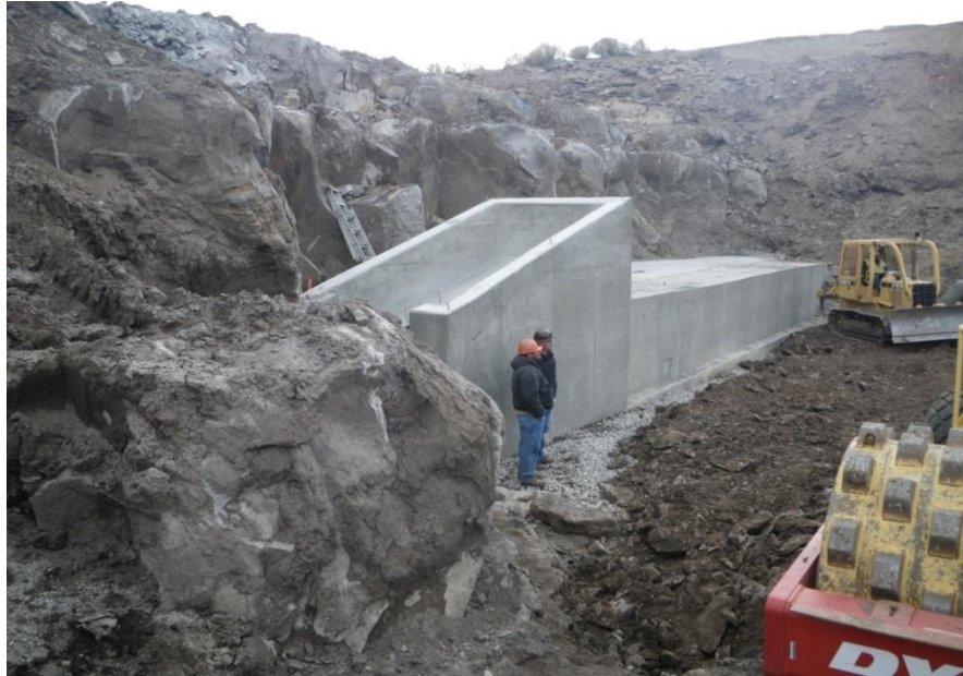
Smith Dam outlet extension and upstream slope rehabilitation.
