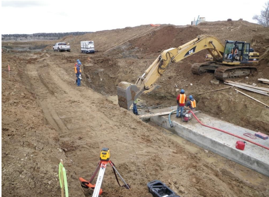
Outlet replacement work at Martin Lake Dam.
