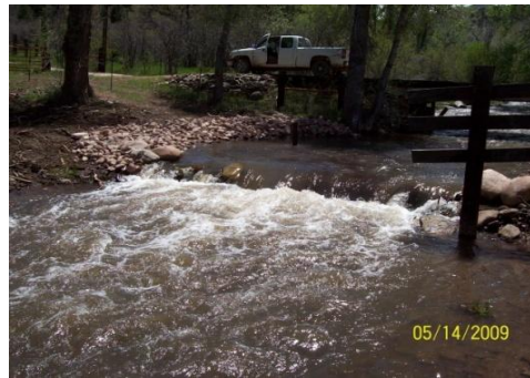
Rock Weir Control Structure
