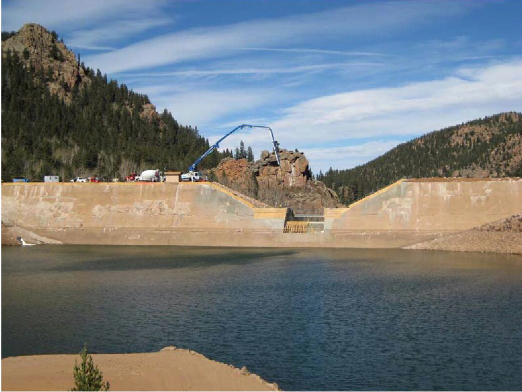
Photo No. 1 – Ogee Crest raising at Big Tooth Dam in the mountains above Manitou Springs.
