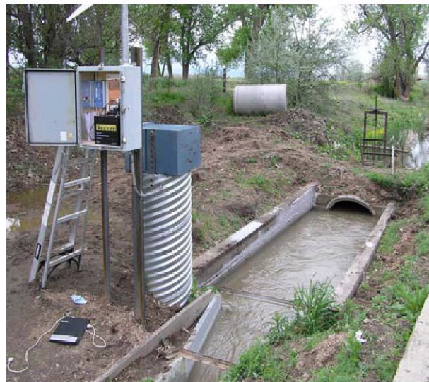
DRGDITCO gage installation
