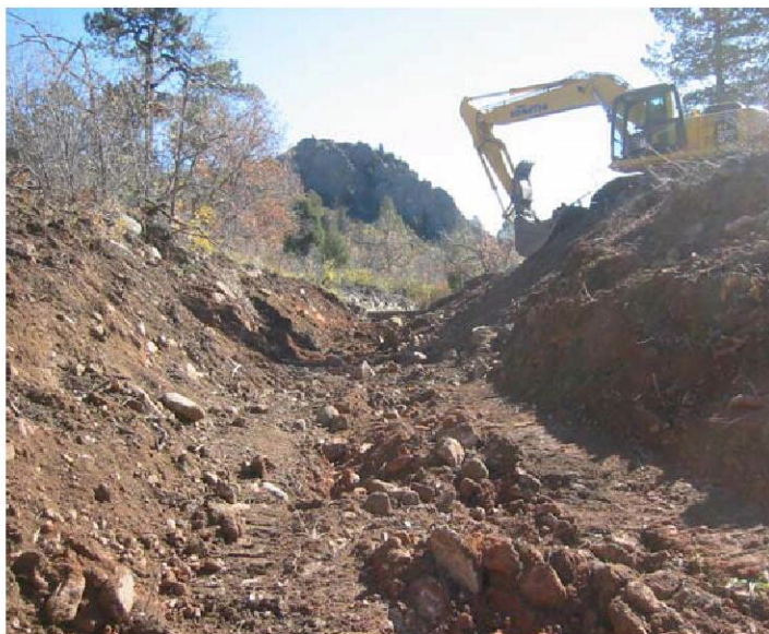
Keeton Dam - Spillway Construction 2006
