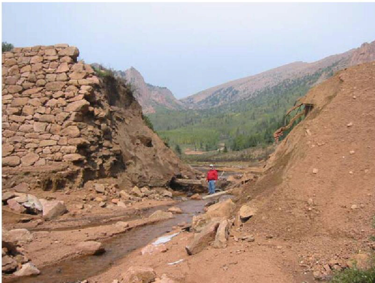
Gillett Reservoir Dam - September 2006
