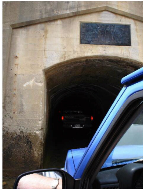
Twin Lakes Tour (going into the tunnel)
