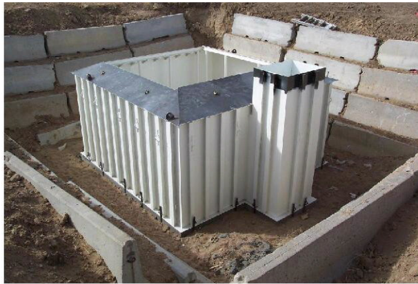
Weighing Lysimeter Construction at Rocky Ford, Colorado February 2006
