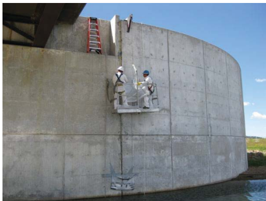
Spinney Dam Spill Repair
