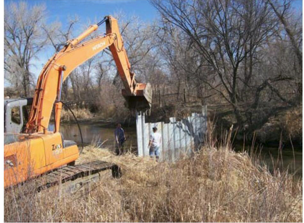
Installing Sheet Piling Control for Springdale Ditch Return Gage
