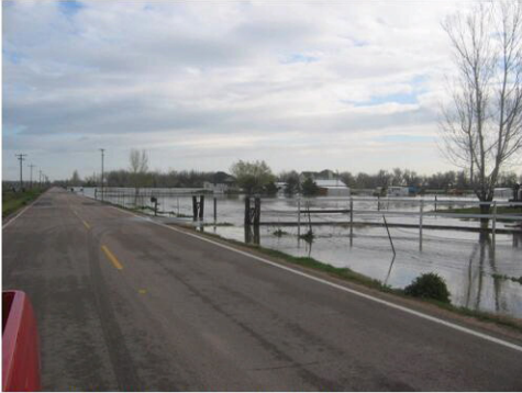
Isolated Flooding in Dist. 2 in April
