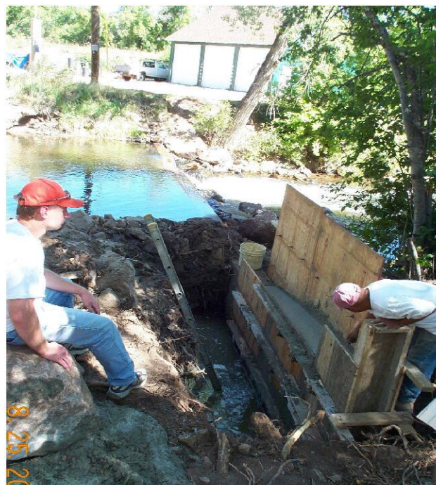
Inspecting Control Work at Bear Cr. At Morrison
