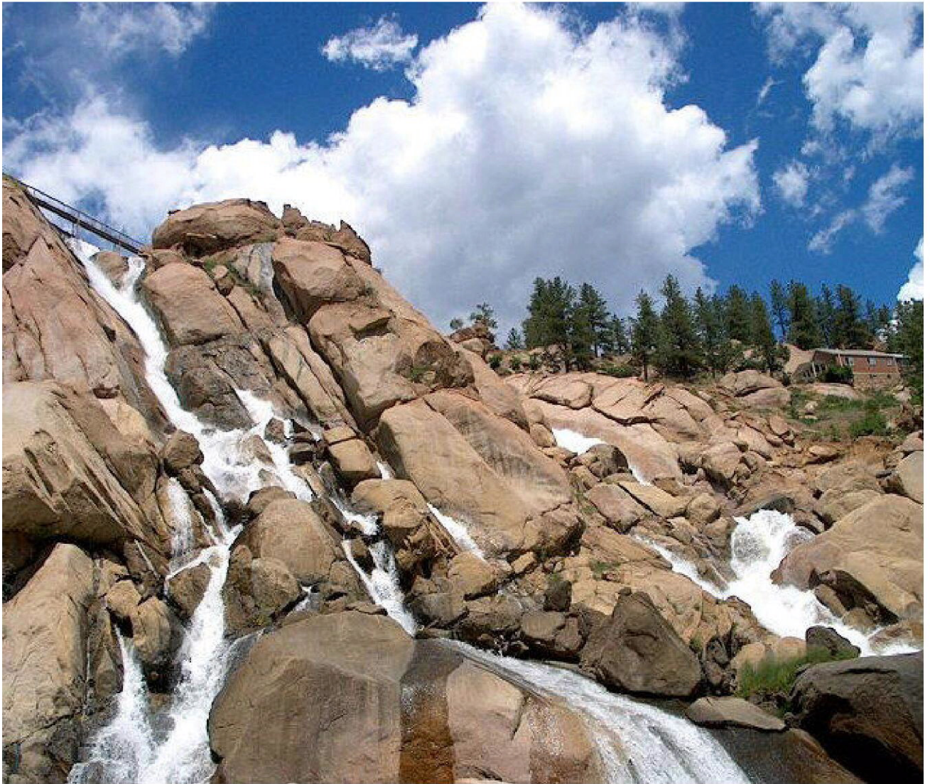
Cheesman Reservoir Spilling (photo by Louis Flink)
