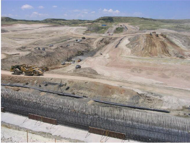
Reuter-Hess Reservoir Construction in Parker
