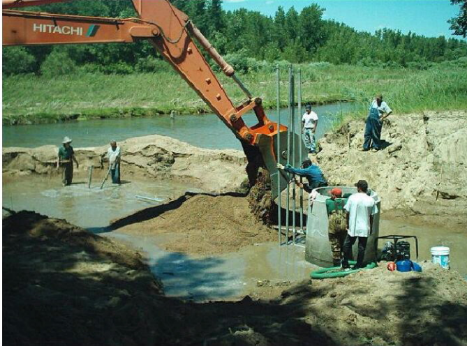
New Gage Installation at South Platte River at Atwood
