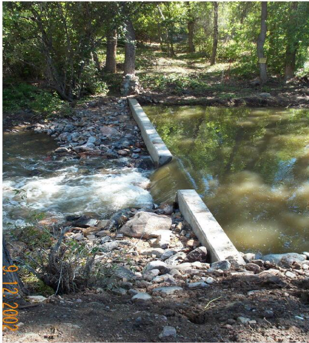
New Bear Creek Control in Operation
