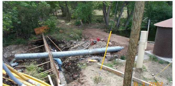
Construction of New Bear Creek Control Structure
