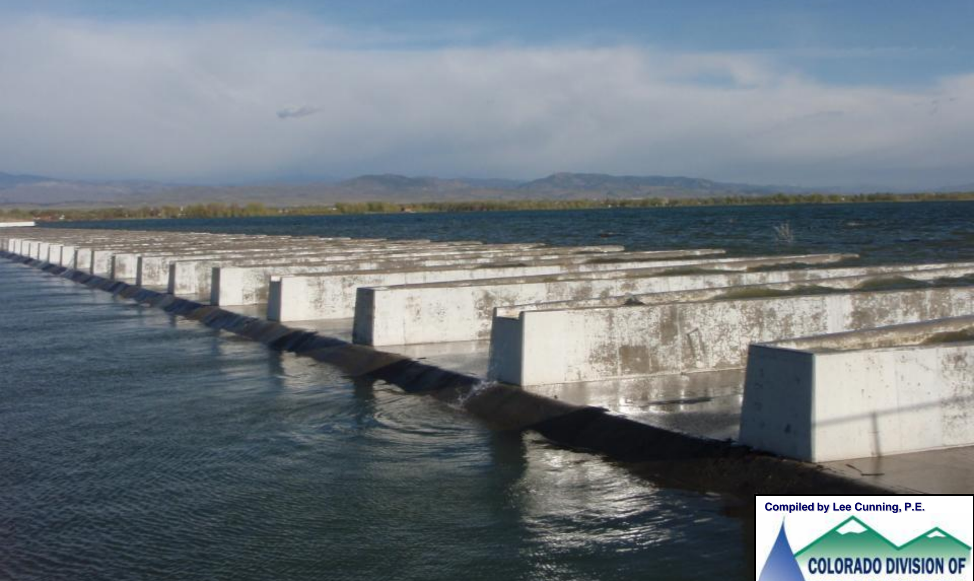
Boyd Lake Spillway Photo by: Jason Smith
