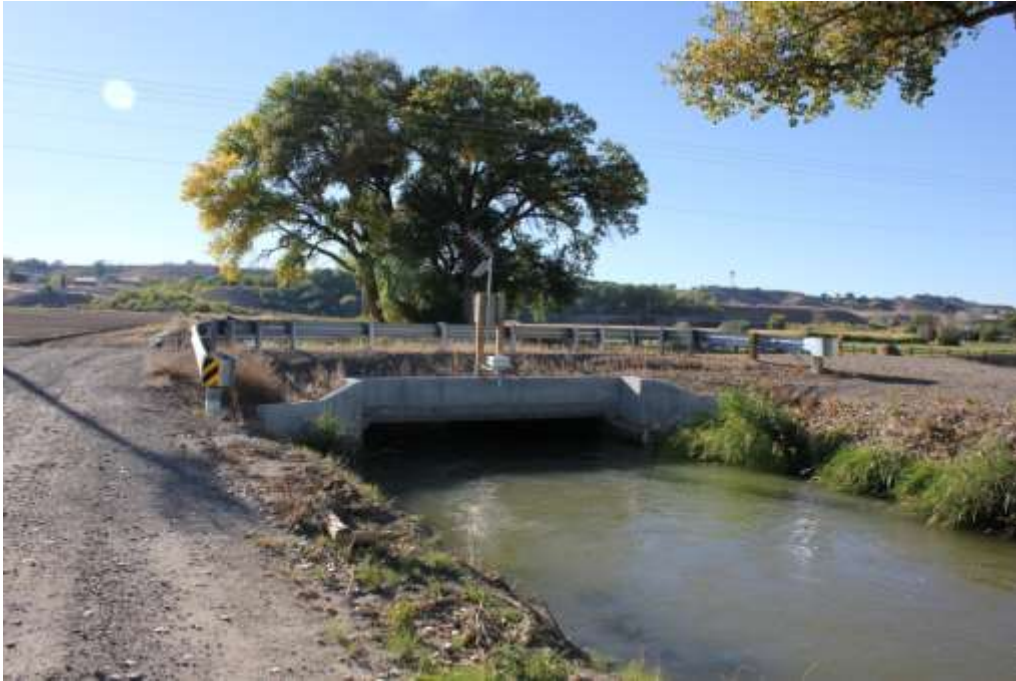
New Ironstone Canal Radar Gage
