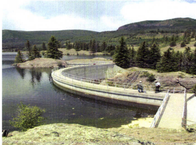
Humphreys Dam, Mineral County Division 3, High Hazard
