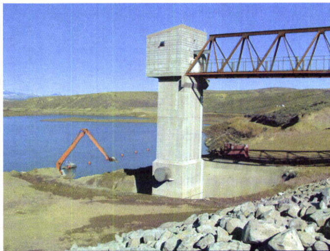
Elkhead Dam Outlet Works Tower Moffat County, Division 6, High Hazard
