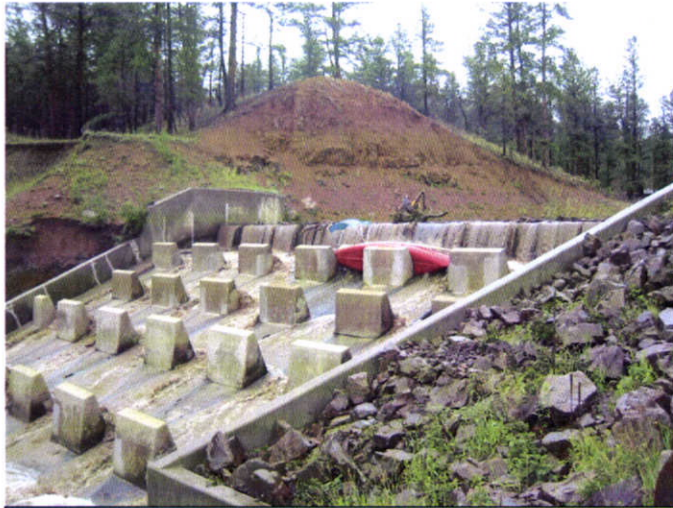
J.O. Hill Dam Emergency Spillway Douglas County, Division 1, Significant Hazard
