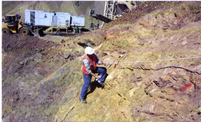
Genesee Dam No. 2, Foundation Inspection Jefferson County, Division 1, High Hazard
