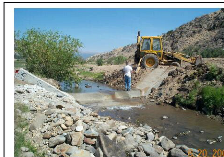
Photo 2 Ramp Flume
