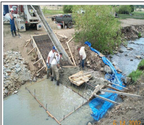
Photo 1 Ramp Flume
