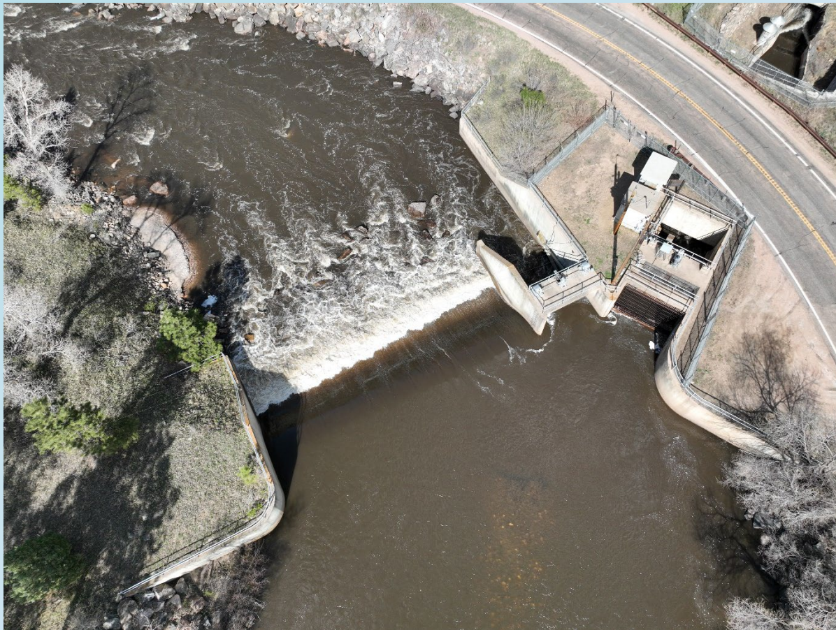
Munroe Diversion Structure, photo by David Bridge
