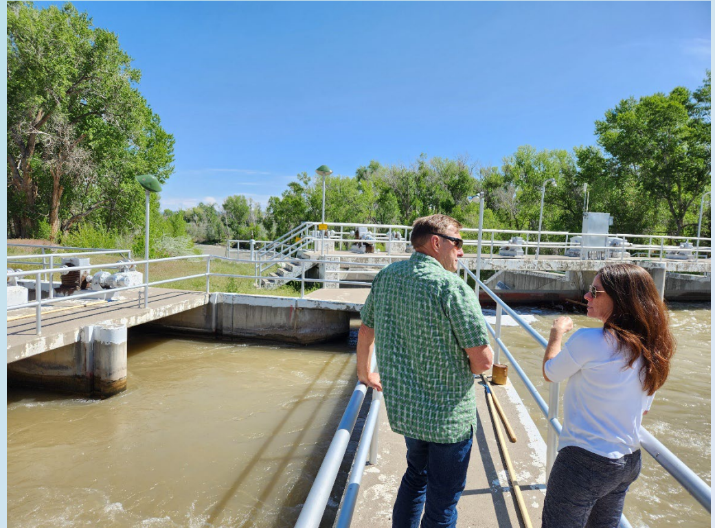
Bob Hurford and Tracy Kosloff at the Montrose and Delta Canal headgate on the Uncompahgre River
