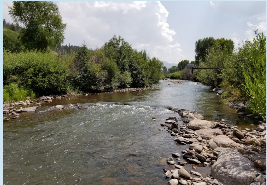
A new cross-vane rock control and radar were installed at Goose Creek near Wagon Wheel Gap. Photo by Jesse Jaminet.
