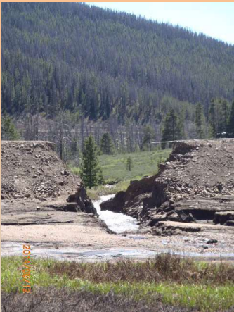
Breached dam at Vagabond Ranch Pond, Grand County Photo by Sue Avre
