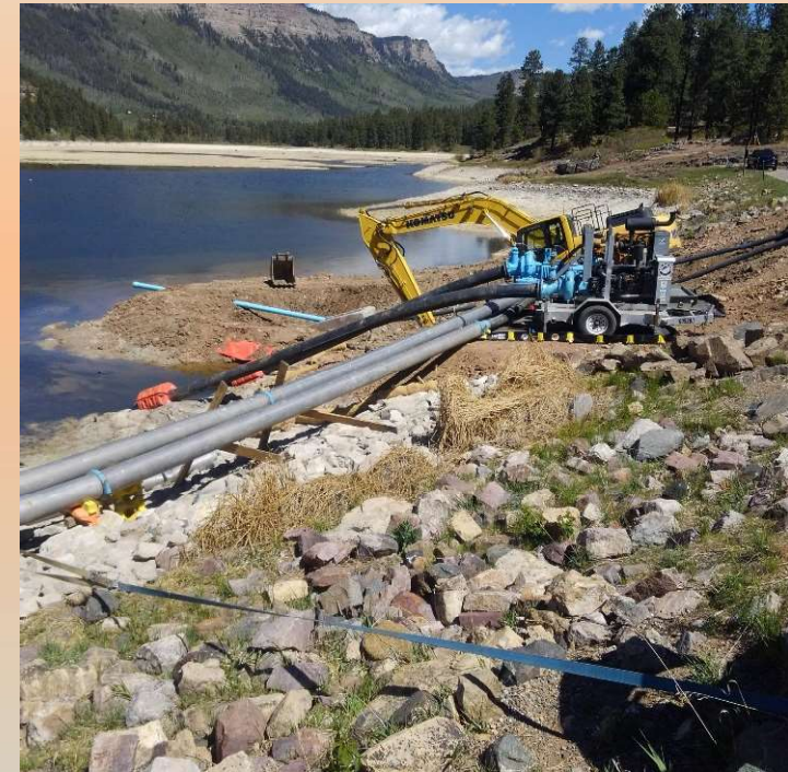
Haviland Lake draw down for outlet repairs. Photo by Jeff Titus
