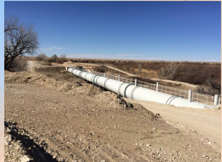
Fort Lyon's Horse Creek Flume
