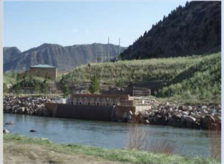
ALP Pumping Plant
