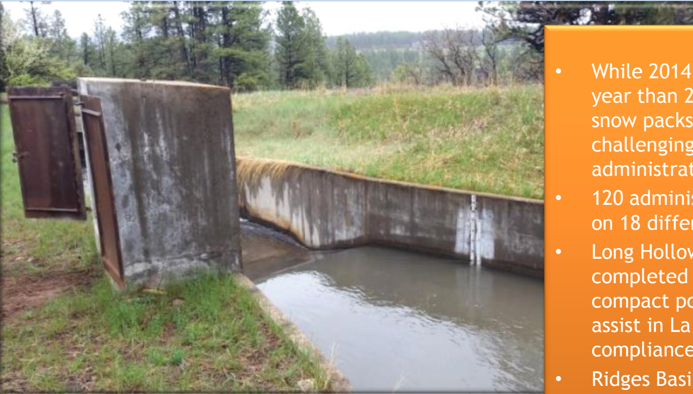
Flume & gauge house, Jackson Gulch Outlet Canal, Mancos, CO
