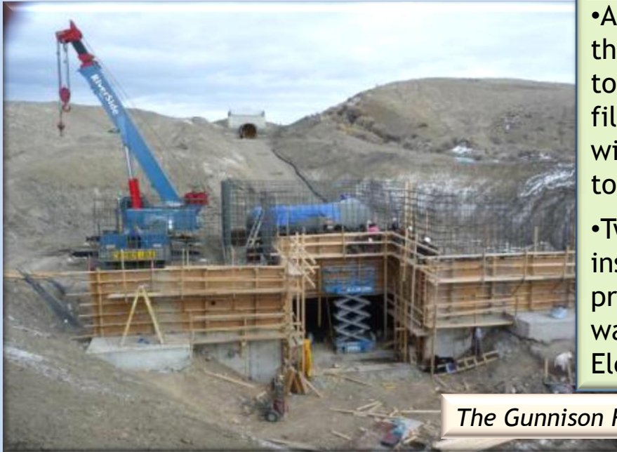
South-Canal Hydroelectric Project Powerhouse & Penstock Drop Structure
