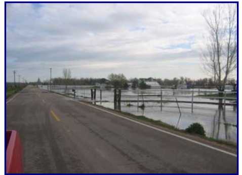
Isolated flooding in Water District 2 in April
