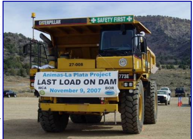
The topping out ceremony for the High Ridges Basin Dam for the Animas-La Plata Project.
