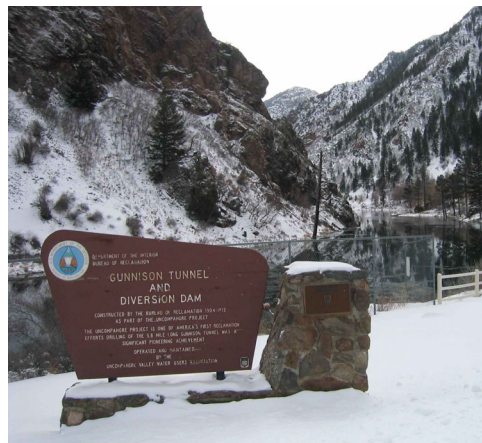
Gunnison Tunnel Diversion in Black Canyon
