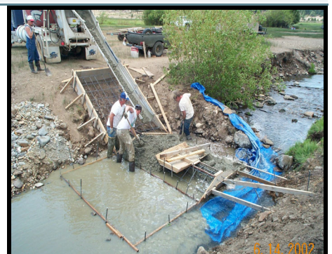
Ramp Flume Installation
