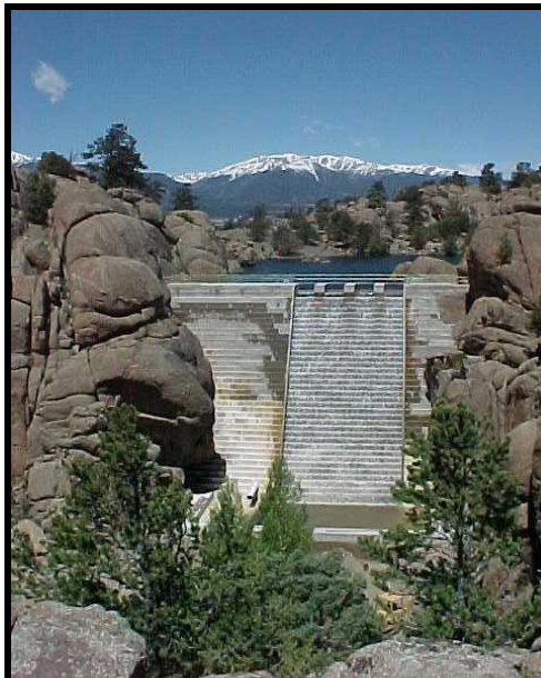
Recently completed Trout Creek Dam, south of Buena Vista, at the bottom of Trout Creek Pass. The dam is 70 feet high with a reservoir storage capacity of 645 acre-feet.
