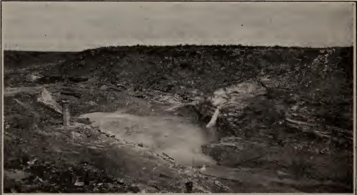
Showing down-stream view of dam-site after failure of dam. The concrete baffle walls, valve tower and remnants of the earth embankment may be seen on the canyon walls.
