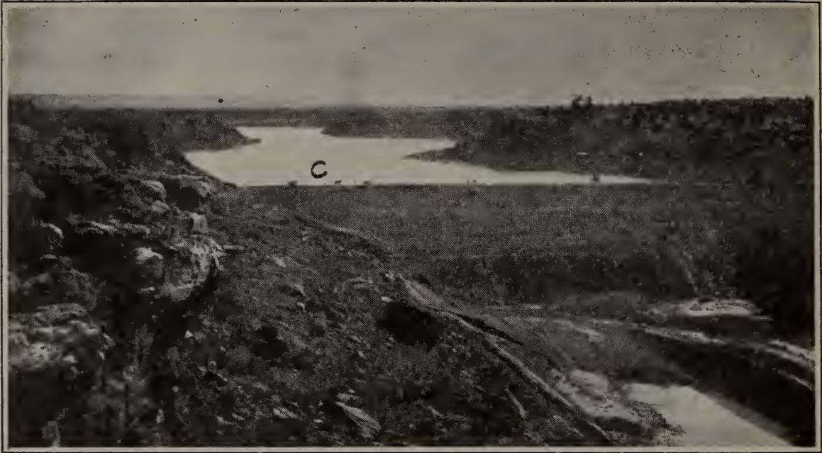
Showing downstream face of Apishapa Dam a few moments before failure on August 22, 1923. Water is seen appearing at right-hand end of dam at point A. Water entering dam at high water line just back of team seen standing on top of dam near C. From this point the water passed diagonally across and lengthwise of the dam to the right-hand end at A.
