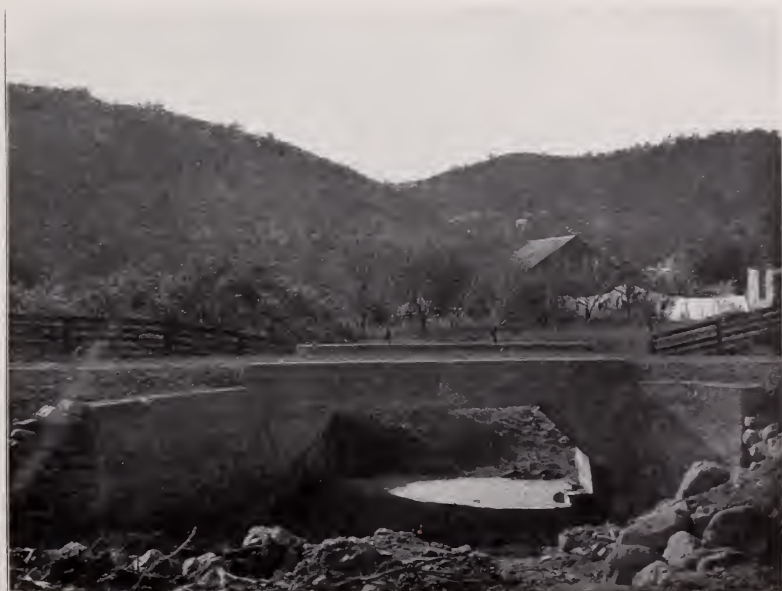
REINFORCED CONCRETE CULVERT BUILT BY CONVICT LABOR ON STATE ROAD NEAR TRINIDAD, COLORADO.
