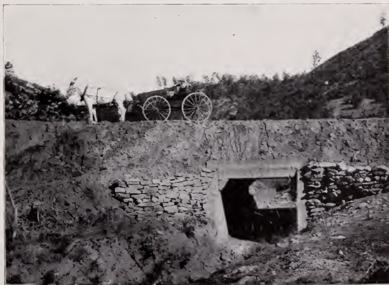
REINFORCED CONCRETE CULVERT UNDER STATE WAGON ROAD. BUILT BY CONVICTS.
