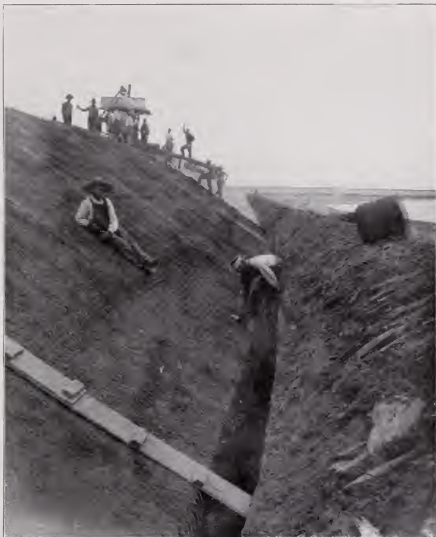
PLACING OF REINFORCED CONCRETE SLOPE PAVING. JACKSON LAKE RESERVOIR. WATER DISTRICT NO. 1.
