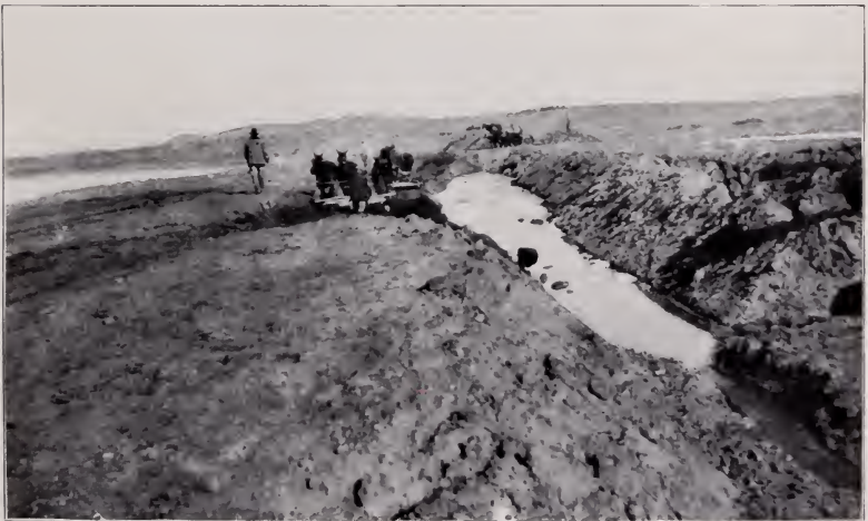
VIEW SHOWING CONSTRUCTION OF ANTERO RESERVOIR DAM AND PUDDLE TRENCH.
