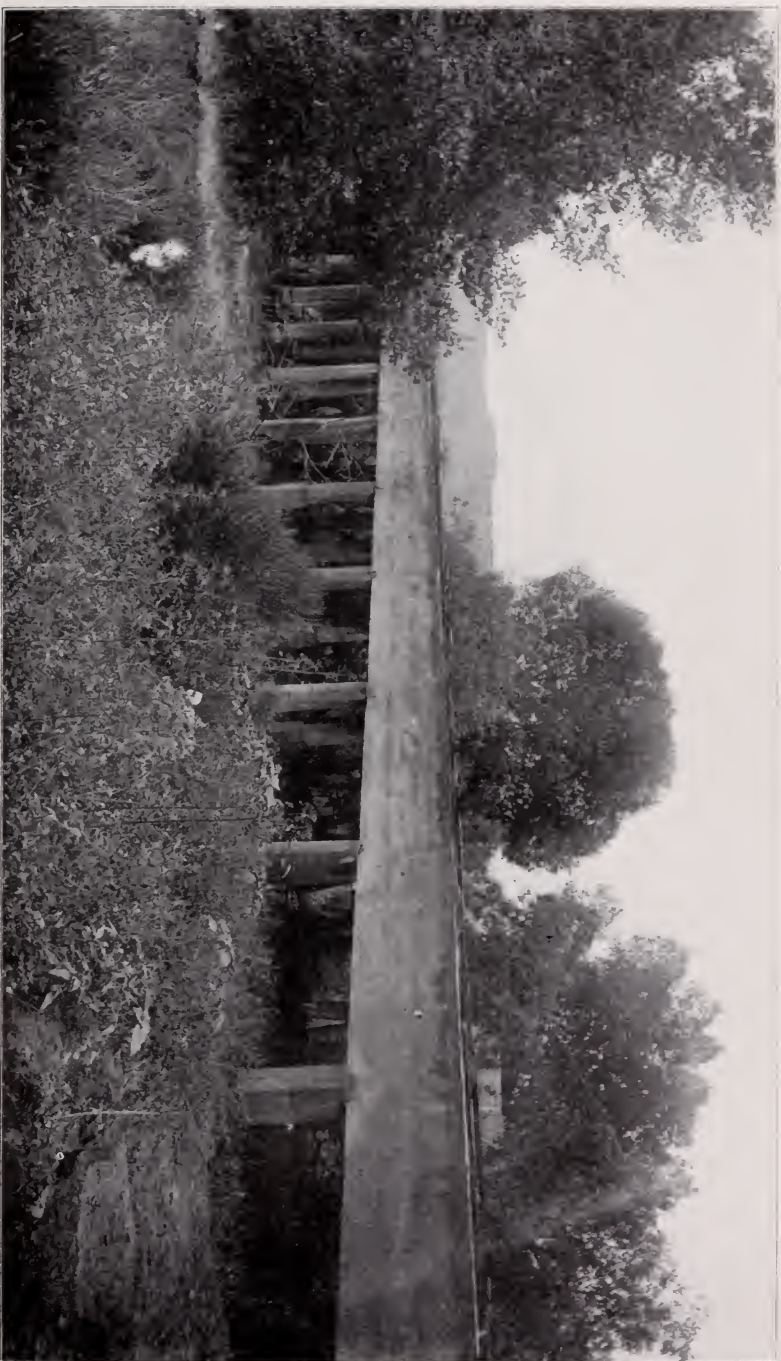
PORTION OF CONCRETE FLUME ON HANDY DITCH, CROSSING DRY CREEK, SIX MILES WEST OF LOVELAND. LENGTH OF FLUME, 768 FEET. SIZE, 3 FEET BY 8 FEET. GREATEST HEIGHT ABOVE THE GROUND, 23 FEET.
