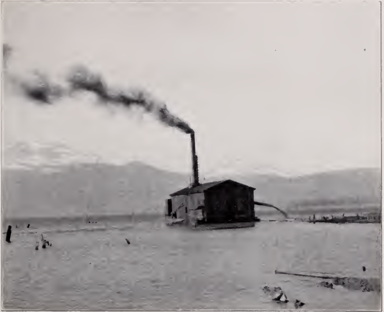
STEAM DREDGE AT WORK ON OUTLET, TWIN LAKES RESERVOIR. WATER DISTRICT NO. 11.
