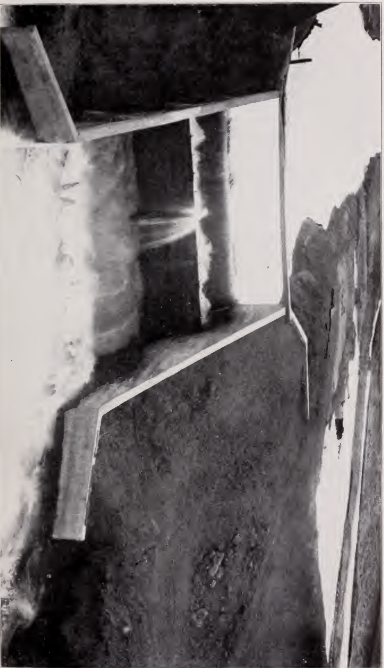
REINFORCED CONCRETE DROP. COMANCHE CANAL, WATER DISTRICT NO. 67. FOUR HUNDRED SECOND FEET OF WATER PASSING.
