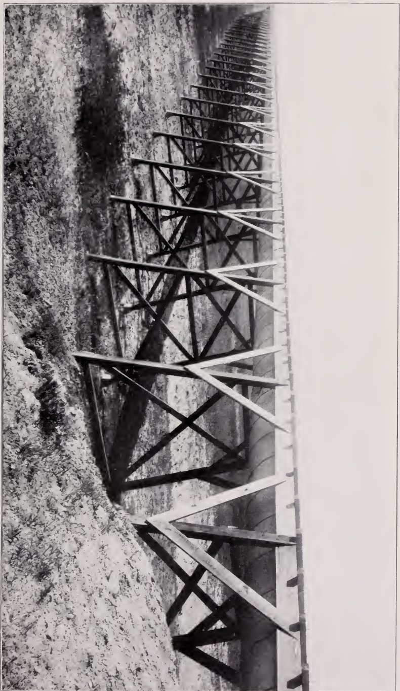
GALVANIZED STEEL FLUME ACROSS CHEYENNE CREEK. WATER DISTRICT NO. 67.
