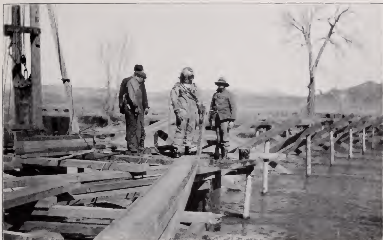
DIVER SINKING TUBES FOR DEL NORTE BRIDGE.
