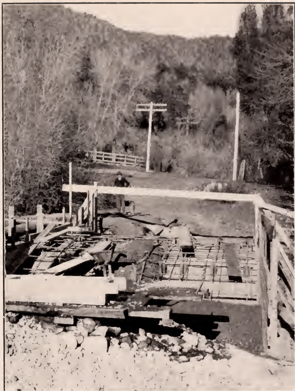
Forms and Steel in Place, Canon Creek Bridge, Garfield County.
