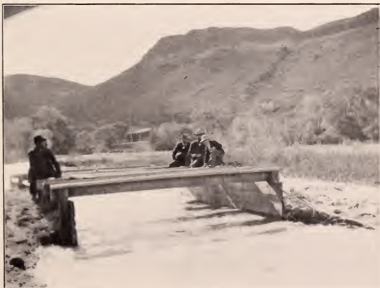
Rating Flume of Rocky Mountain Ditch, Near Golden, Water District No. 7.
