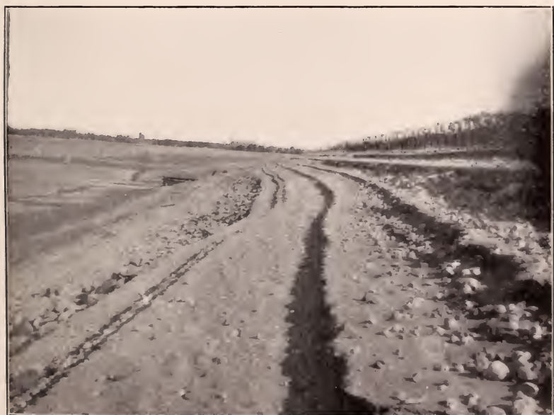
Showing Effect of Wave Action on Unprotected Embankment—Cache La Poudre Reservoir, Water District No. 3.
