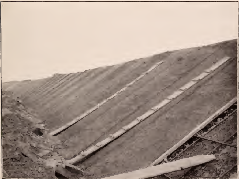
Completed Reinforced Concrete Slope Protection, Terry Lake Reservoir, Larimer County.
