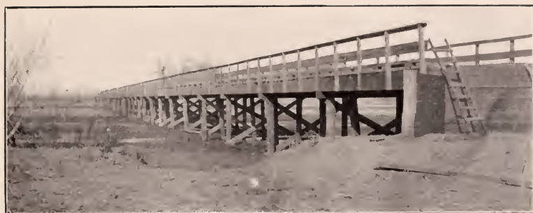
Pile Bridge, Arkansas River, Morse Siding, Prowers County.
