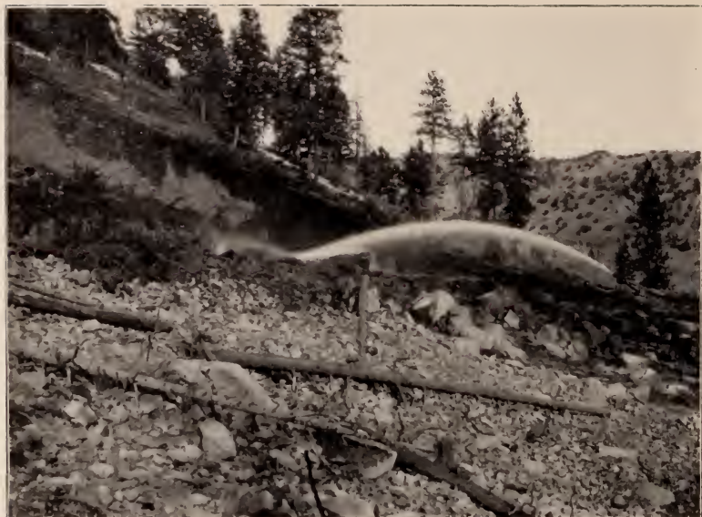
Hydrauliclicking Materials for Inside Slope of Terrace Reservoir, Conejos County.
