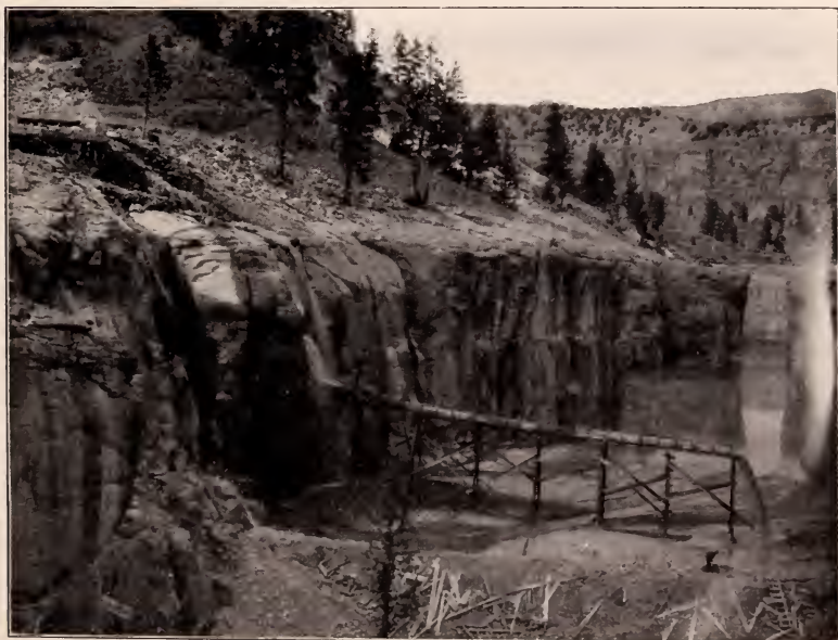
Depositing Material Outside Slope of Reservoir—Terrace Reservoir, Conejos County.
