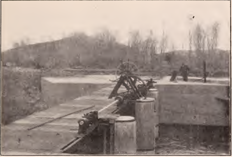
Lifting Apparatus for the Head Gates of Larimer County Ditch, Cache la Poudre River, Larimer County.
