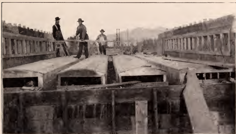
Forms for Reinforced Concrete Bridge, Alamosa.
