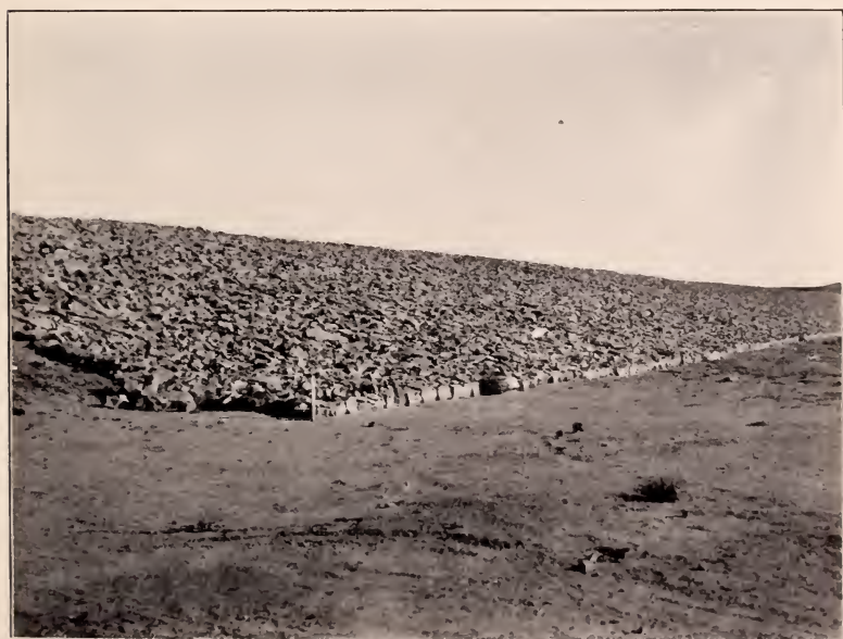
Slope Paving, Julesburg Reservoir, Sedgwick County.
