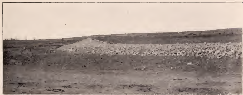
Shale Surfacing Bent County Road, Near Las Animas.
