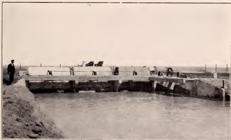
Reinforced Concrete Radial Check Gates, Amity Canal at Big Sandy Creek, Water District No. 67.
