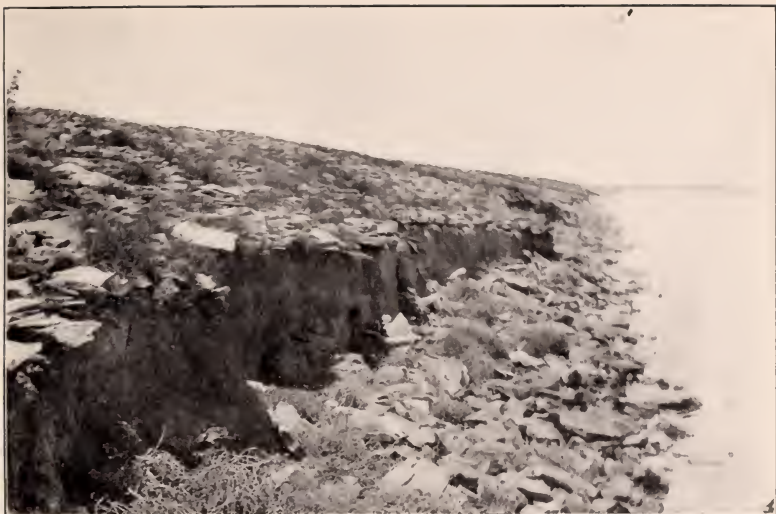
Effect of Wave Action on an Earth Dam.
