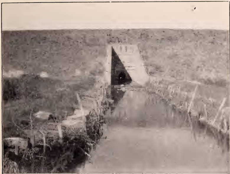
Showing Method of Riprapping Outlet Channel, Cache La Poudre Reservoir, Water District No. 3.
