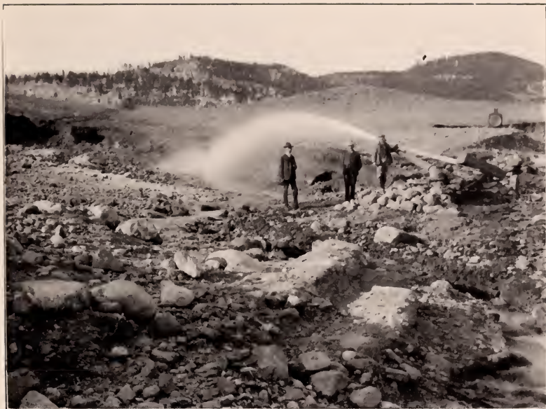
Hydraulicking Material for Outside Slope of Terrace Reservoir, Conejos County.
