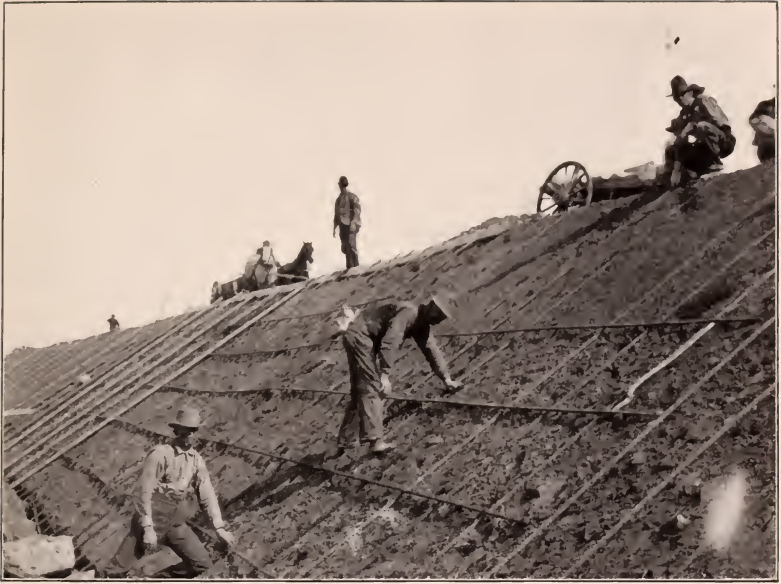
Placing Steel Bars, Reinforced Concrete Slope Protection, Terry Lake Reservoir, Larimer County.
