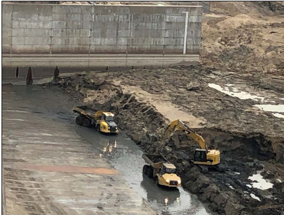
Sediment removal from the John Martin Reservoir stilling basin.
