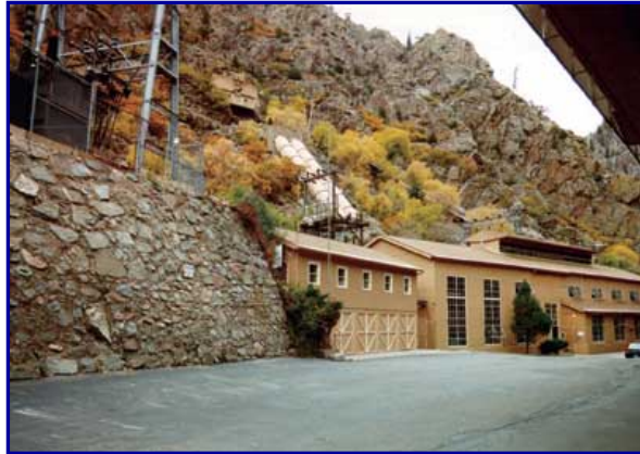
Shoshone Hydroelectric Power Plant. Picture courtesy of the Colorado River Conservation District
