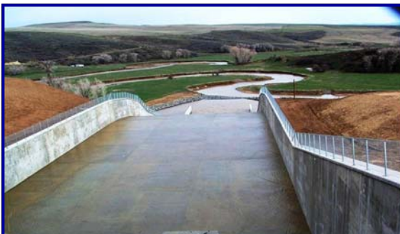
Spillway on enlarged Elkhead Reservoir
