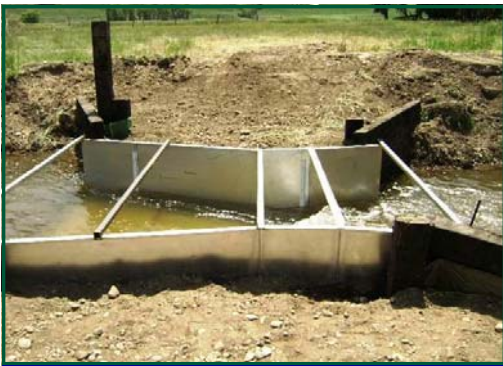
New flume on the Deep Cut Ditch
